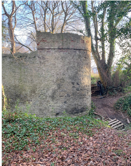
External view from outside the north west corner of the walled garden showing the curved corner of the mid 19th century corner tower.
