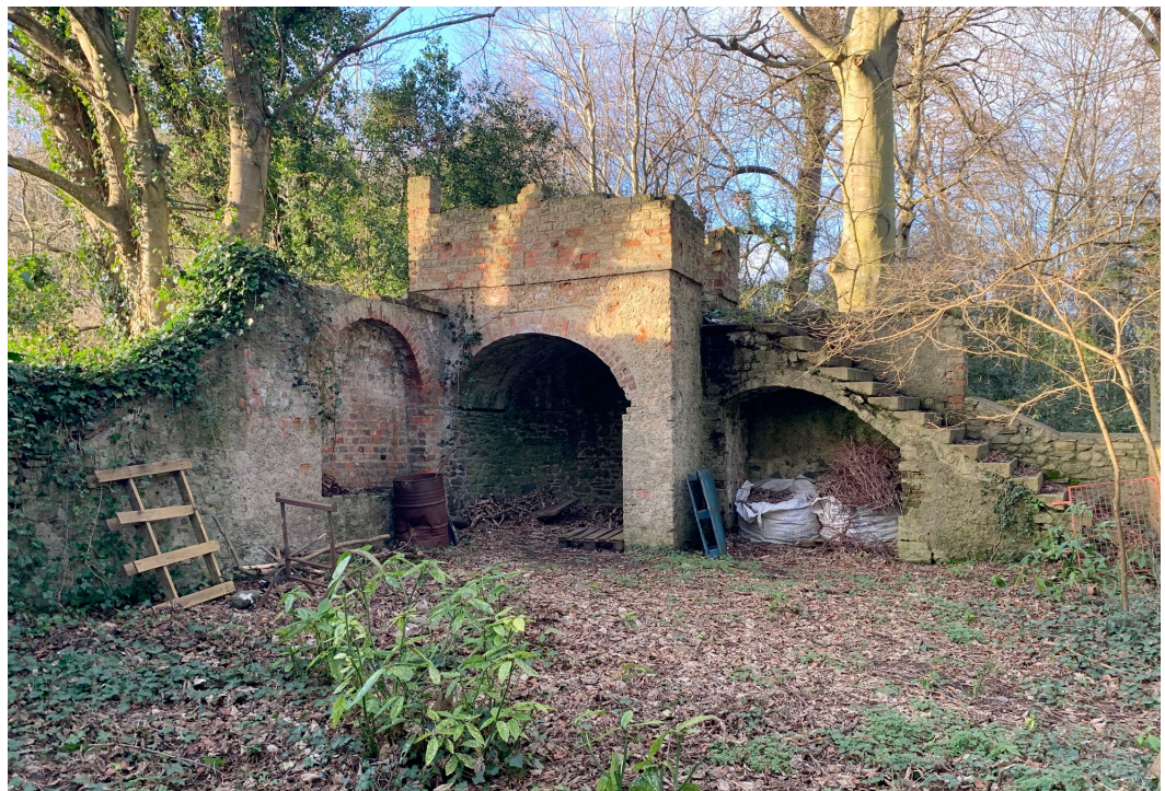
Internal view of the corner tower at the north western corner of the walled garden - this and the equivalent corner tower at the south west corner to be stabilised and repaired so that they are safe and conserved as a landscape feature within the walled garden.
